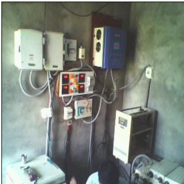
Figure 4 : Charge Controller setup
