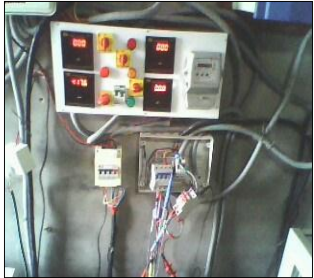
Figure 2: Vertical Wind Turbine Generator Setup Figure 3: Generator output connection
